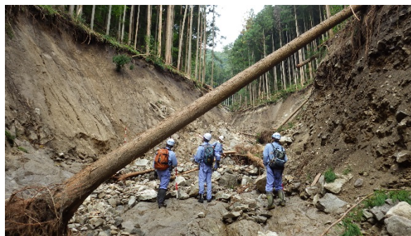
Photo: Debris flow disaster investigation (Nikko-shi, Tochigi)
