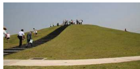
Photo 3. Example of Miniature Hill Created to Provide Safe Haven for Tsunami Evacuees (Central Park in Kamisu City)
