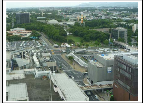
Photo 1. Underground TX Tsukuba Station and Traffic Square
