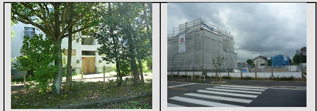
Photo 2. Former Takezono 3-Chome National Public Officer's Housing Complex and Private Sector Housing under Construction at the Vacant Lot of the Former Housing Complex
