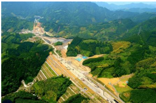
Photo 2 Large scale embankment
