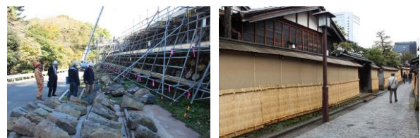
Photo (left): Stone wall restoration of Sendai Castle, (right): Clay wall restoration with straw matting by students of the Kanazawa Institute of Traditional Crafts
