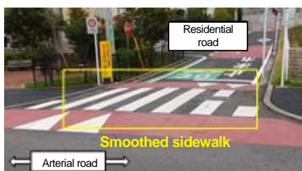
Photo 2 Smooth sidewalk (Raising the sidewalk across the intersection to form a level difference in the traffic lanes)
