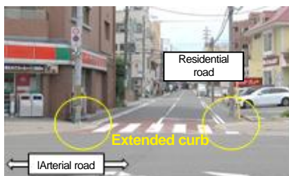
Photo 1 Intersection curb extension (extending sidewalks at an intersection to narrow the space for cars to enter the residential road)
