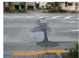
Photo 2. Characteristic Joint Damage on Concrete Pavement and State of Repair
