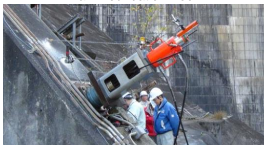
Figure 2. Lift-off Test Conducted in Trial Inspection
