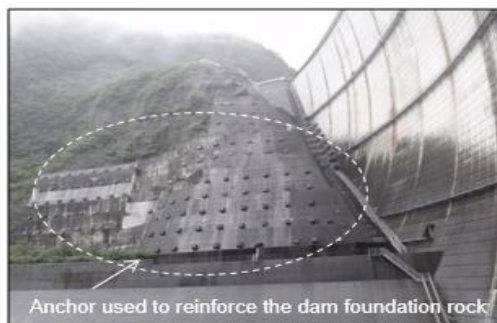
Figure 1. Example of Anchor Used to Reinforce the Dam Foundation Rock
