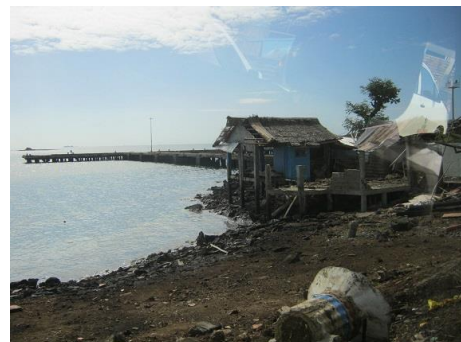
Photo-1 Damage of port in Philippines caused by Typhoon 1330 (Haiyan) (Port of Estacia) 1),2)
