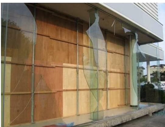
Photo 1: Damaged glass screen by earthquake after its damage
