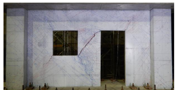
Photo 3: Damage conditions at story deformation angle 1/100\text{rad}
