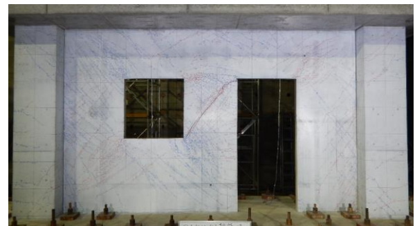
Photo 2: Damage conditions at story deformation angle 1/200\text{rad}
