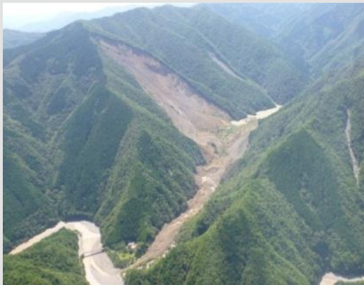
Figure 1. Deep-seated Landslide Generated in Kii Peninsula in 2011
