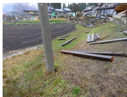
Photo 2: Stone walls and power poles damaged southward
