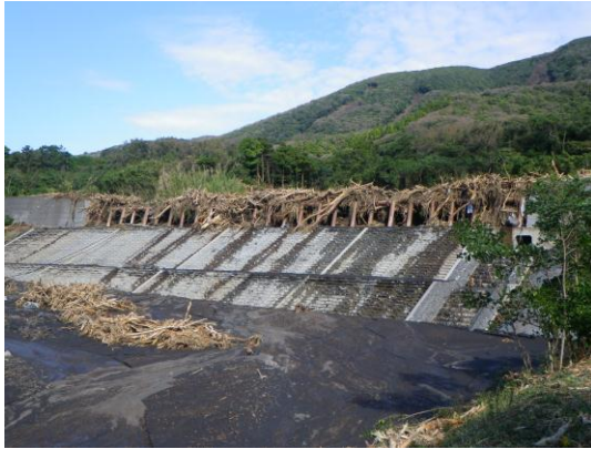
Photo 3 Capture of debris flows and driftwoods by a sediment-related disaster prevention facility along Okanesawa River
