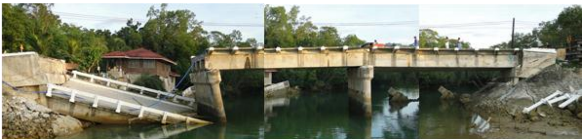
Photo: Damage to Moalong Bridge (Built in 1982)
