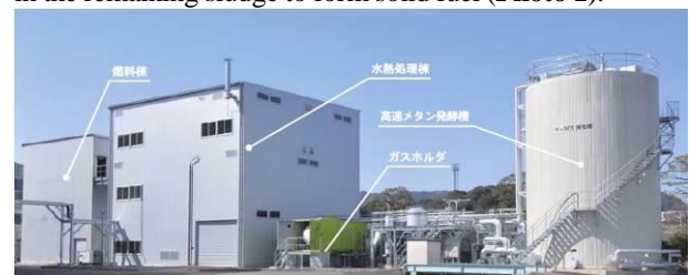
Figure 1: Appearance of Verification Facility (Nagasaki Eastern Sewage Treatment Facility)
