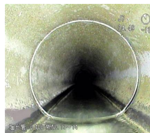
Photo 1: Example of Flatness
