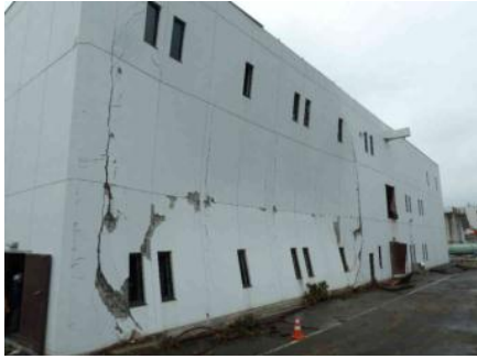
Photo 1 Damages on building by tsunami
