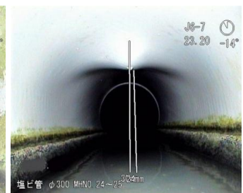
Photo 2: Example of Deformation
