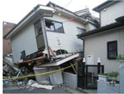
Photo 2: Collapse of upper structure in timber housing
