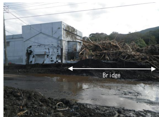
Photo 2 Blockage of driftwoods at Motomachi Bridge
