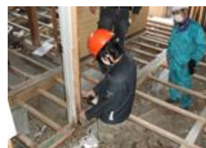
Photo 2: Implemented situation of degradation survey
