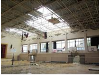
Photo 1: Damage in educational facility A Gymnasium
