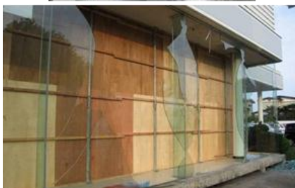
Photo: Damage assumed to be affected by out-of-plane vibration.
