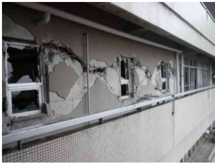
Photo 2 Damages on non-structural wall by earthquake
