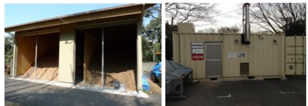
Photo. Use of Branches Pruned from Park Trees to Heat Park Facilities (Oi Pier Central Seashore Park: Tokyo) (Left: Chip dryer using solar heat, right: boiler)
