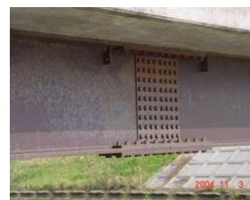
Photo 1. Example of a steel bridge high strength bolted friction joint
