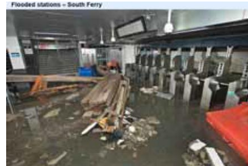
Photo: Flooded Subway Station (Source: Metropolitan Transportation Authority)
