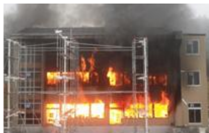
Photo 2: Fire spread to the 3rd floor
