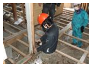
Photo 2: Implemented situation of degradation survey
