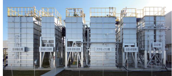
Figure 4: Appearance of Verification Facility (Kumamotoshi Eastern Purification Center)
