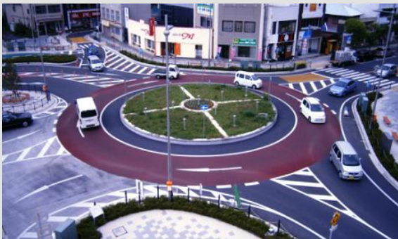
Photo 1. Example of construction (Hitachi City in Ibaraki Prefecture)
