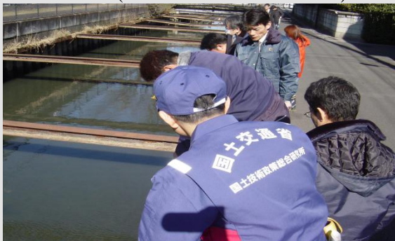
Figure: Sheet-Pile Revetment Deterioration Survey by River Structure TF
