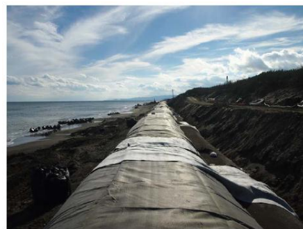
Photo 2: Sand Dune Scarp Control Works Adopted or Miyazaki Coast
