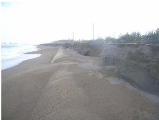
Photo 1: Sand Dune Scarp Control Works Fit for
