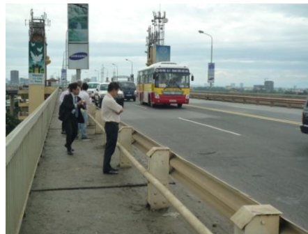
Photo 2. Technicians from the NILIM and PWRI etc. Inspecting Pavement at the Thang Long Bridge in Vietnam
