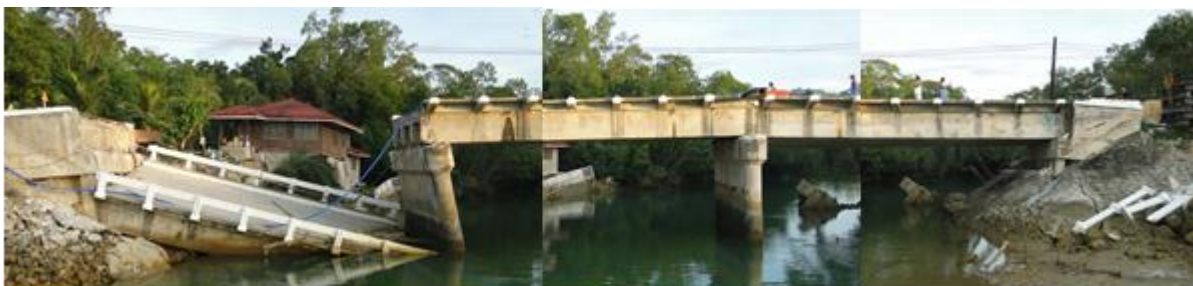
Photo: Damage to Moalong Bridge (Built in 1982)
