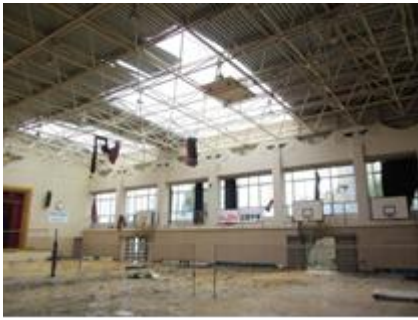
Photo 1: Damage in educational facility A Gymnasium
