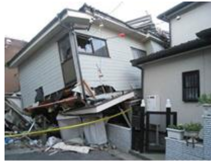
Photo 2: Collapse of upper structure in timber housing
