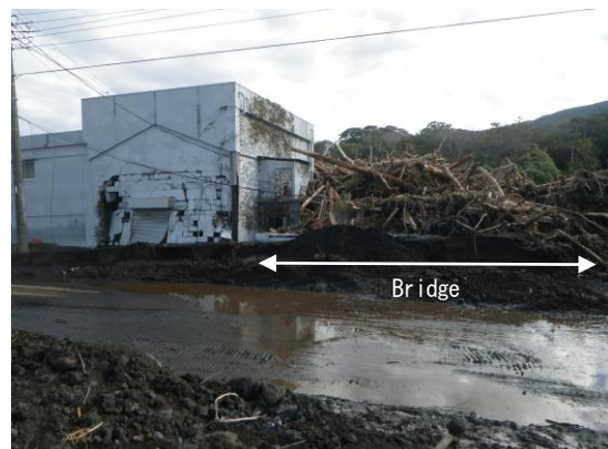
Photo 2 Blockage of driftwoods at Motomachi Bridge
