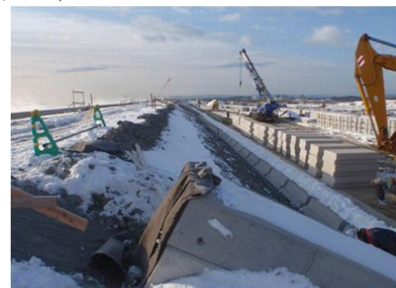
Photo: Laying works of cutout blocks
