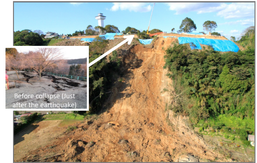
Photo 1 Example of the slope that has collapsed by the rainfall after to the Great East Japan Earthquake, 2011(provided by Tochigi Pref.)
