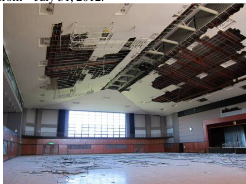
Photo: An example of the ceiling falling off damage in a gymnasium
