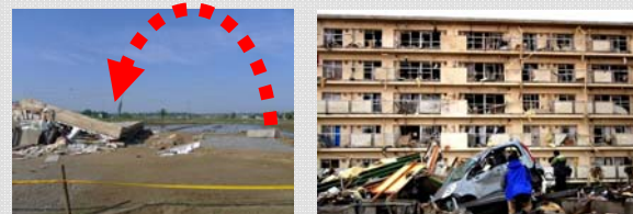
Overturned building (Photo-1) Wind pressure of the tornado and hit by flown objects (Photo-2).
