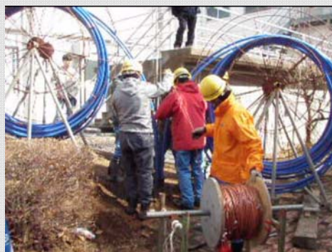
Photo 1 Installation of the U-tubes
