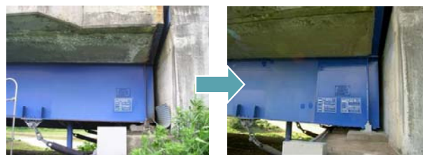
Fig. 2. An example of a bridge with considerable corrosion at the ends only.
