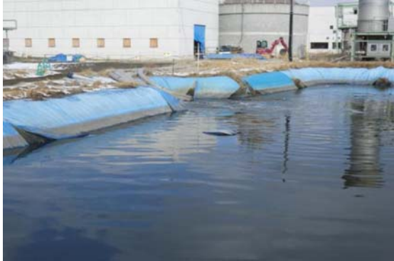
Photo Example of emergency restoration works (Temporary sedimentation tank constructed by rough digging)
