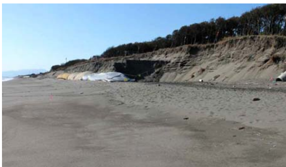
Photo 1 Preventive effects to the earth fill on the back
