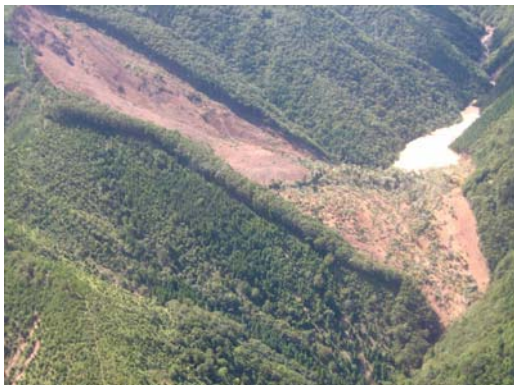
Photo 1. River Course Blockage at Nagadono Valley in Totsukawa Mura in Nara Prefecture
