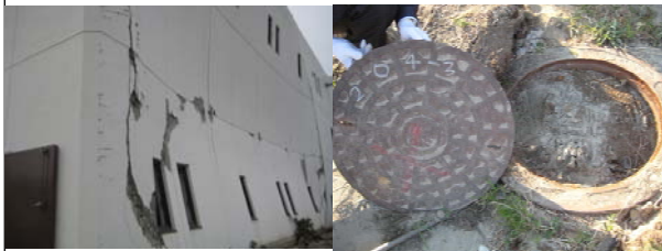
Figure 1. View of Damaged Sewage Facilities
