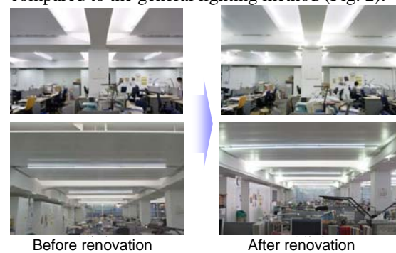
Figure 1. Task and ambient lighting before and after renovation
