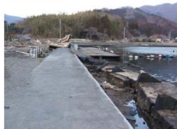
Photo 1. View of Damage to a Seawall (by the Backwash)
