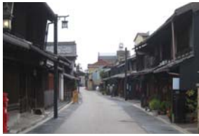
Transformer is in a back alley, eliminating above ground equipment.
