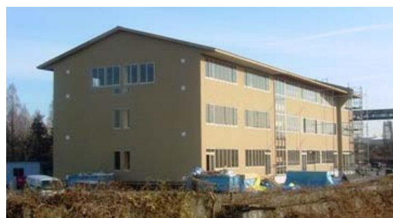
Photo 1. The Experimental Three-story Wooden School Building
