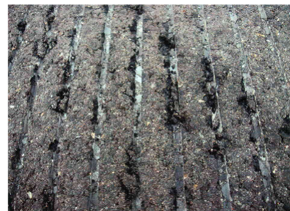
Figure 2. Failure of grooves
