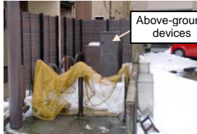
Above-ground equipment installed in the local garbage disposal site
