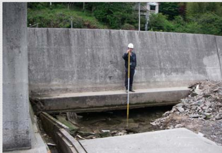
Photo: A field survey in progress
