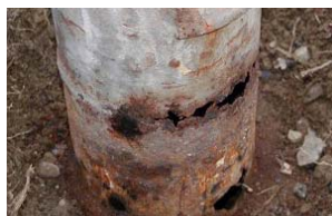
Photo 1. Column Base Corrosion Covered by Paving
