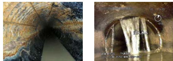
Photo 1. Examples of failed sewers
