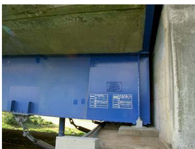
Photo 2. Trial Execution on an Actual Bridge
