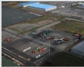
Photo 1: Scattered containers (provided by Japan Coast Guard)
