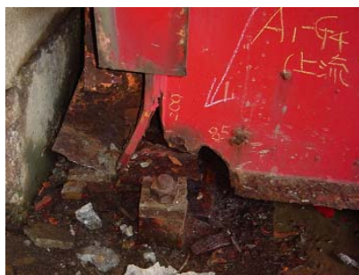
Photo 1. Example of Girder Edge of Main Girder Showing Local Corrosion
