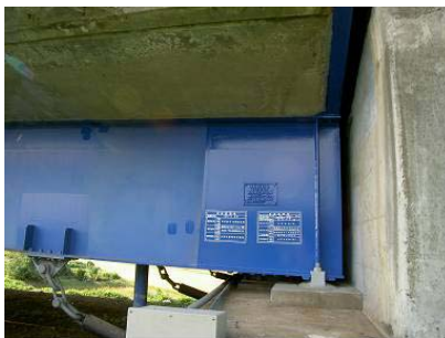
Photo 2. Trial Execution on an Actual Bridge
