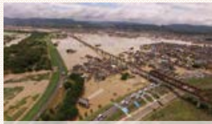
Levee breakage due to heavy rain in July 2018
