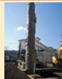
Removing an existing pile
