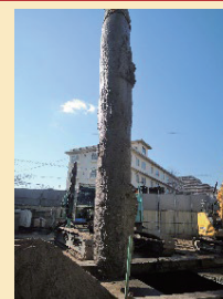
Removing an existing pile
