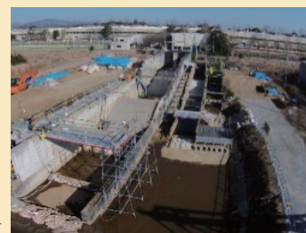
Construction of an experimental channel to enable the overflow experiments necessary to study the development of tenacious river levees.
