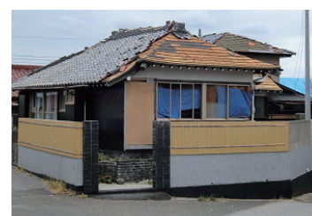
Example of damage to tile roofs caused by a typhoon (Typhoon Faxai in 2019)
