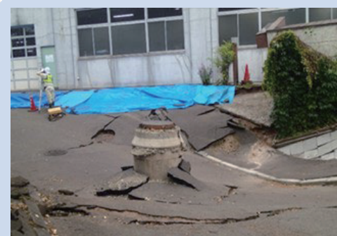
Manhole floating from liquefaction
