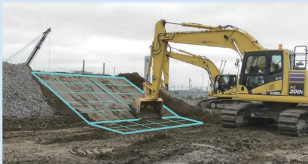
Workmanship management using the recorded data of the cutting edges of construction machinery
