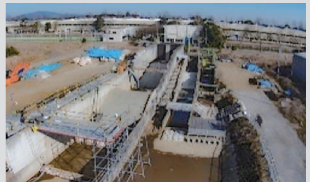
Construction of an experimental channel to enable experiments using a full-scale embankment model (approximately four-meter high)
