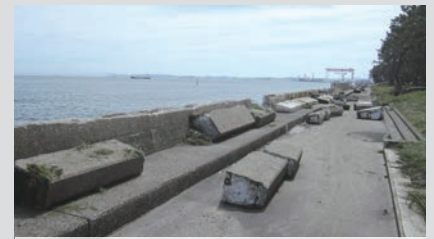
Damage to the seawall caused by the tidal waves of Typhoon No. 15 (Faxai) in 2019
